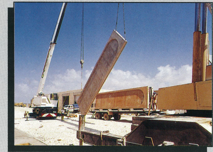
Erection of Wall Panels
