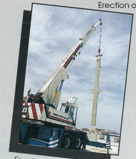
Erection of Columns
