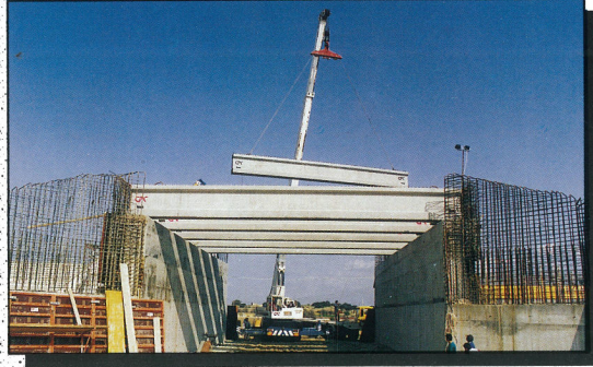
Prestressed I-Beams at new Air Terminal Bridge
