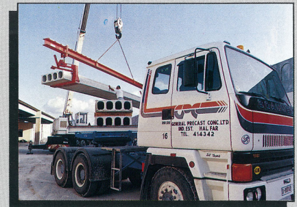
Erection of Drycast Slabs
